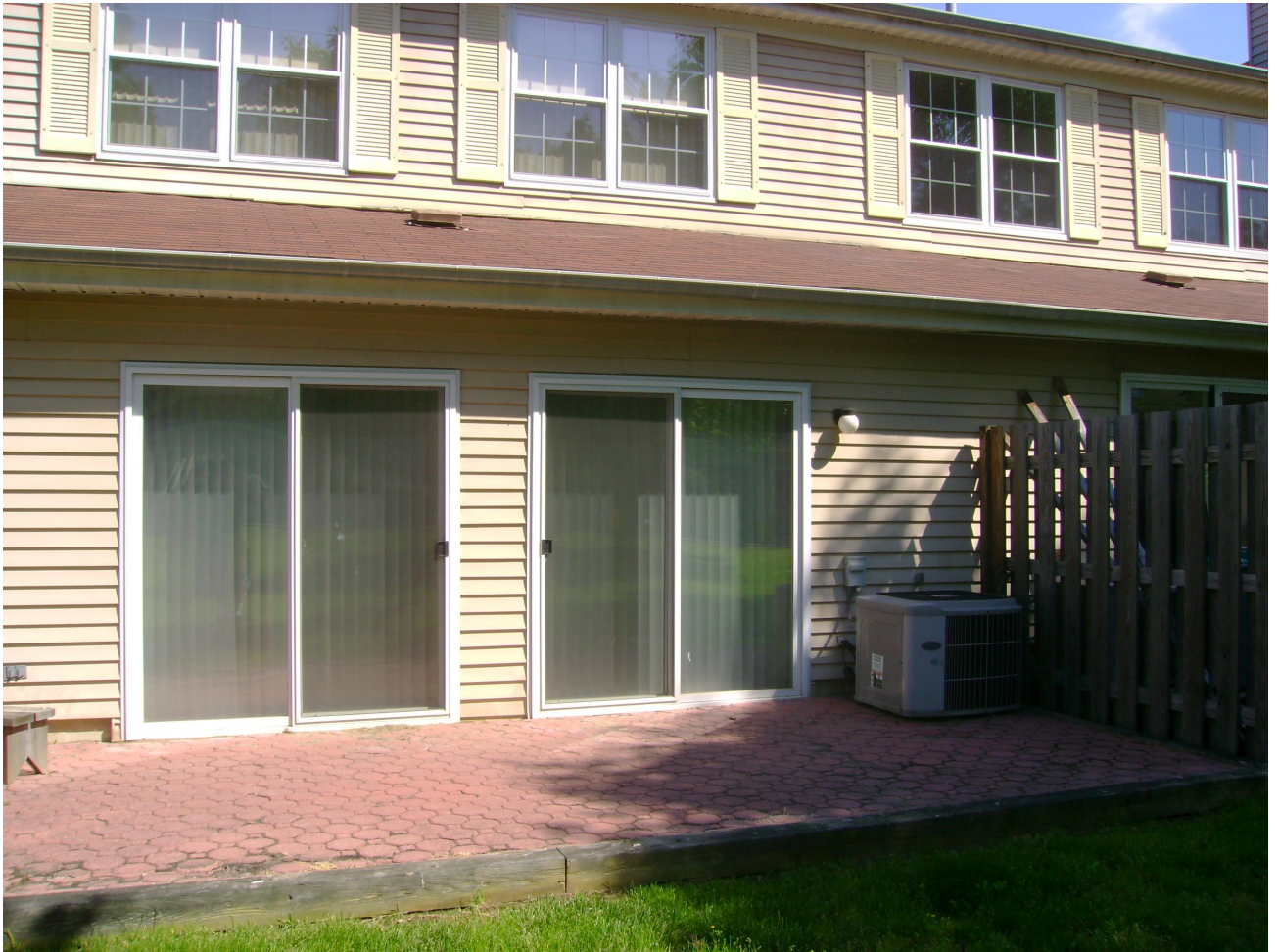
An example of a conforming patio.
